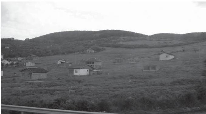
Figure 7. New Houses Built without Permission from Regulatory Authorities, Kavaklija Neighborhood, Dupnitsa
