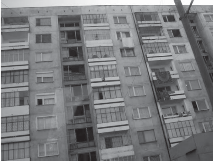
Figure 27. Housing Estate in Stolipinovo Neighborhood, Plovdiv
