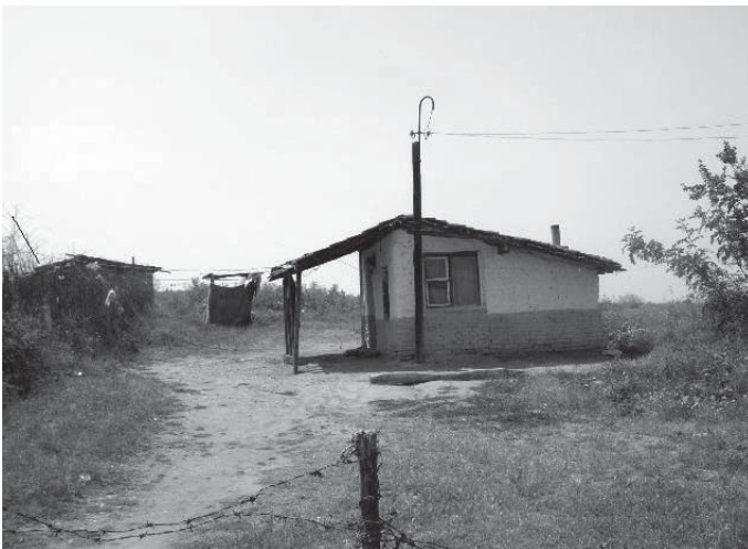
Figure 1. House Connected to the Electricity Grid, Lagera Roma Neighborhood, Simeonovgrad
