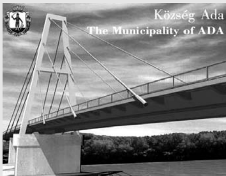
Figure 3. Bridge on the River Tisa
